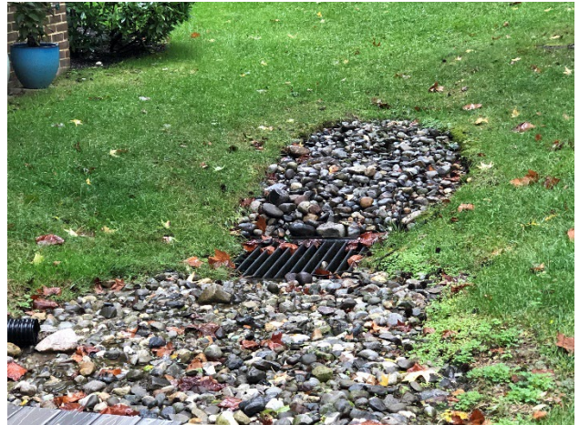
Photo 4. Existing inlet to be converted to proposed overflow.
